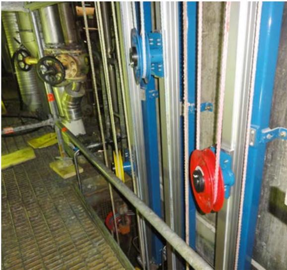
Thanks to the tensioner's compact footprint, it was possible to position the unit in a very tight area. The flexible design also meant an offset mounting bracket could be utilised to maintain the correct alignment.
