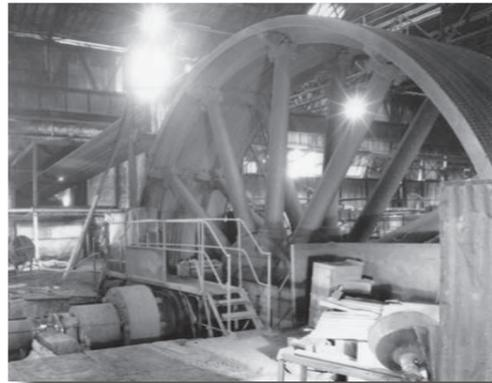
A rolling mill drive at Llanely steel works circa 1907. It used forty 237 foot ropes on the sheet steel drive and four 78 foot ropes to drive a compressor.
